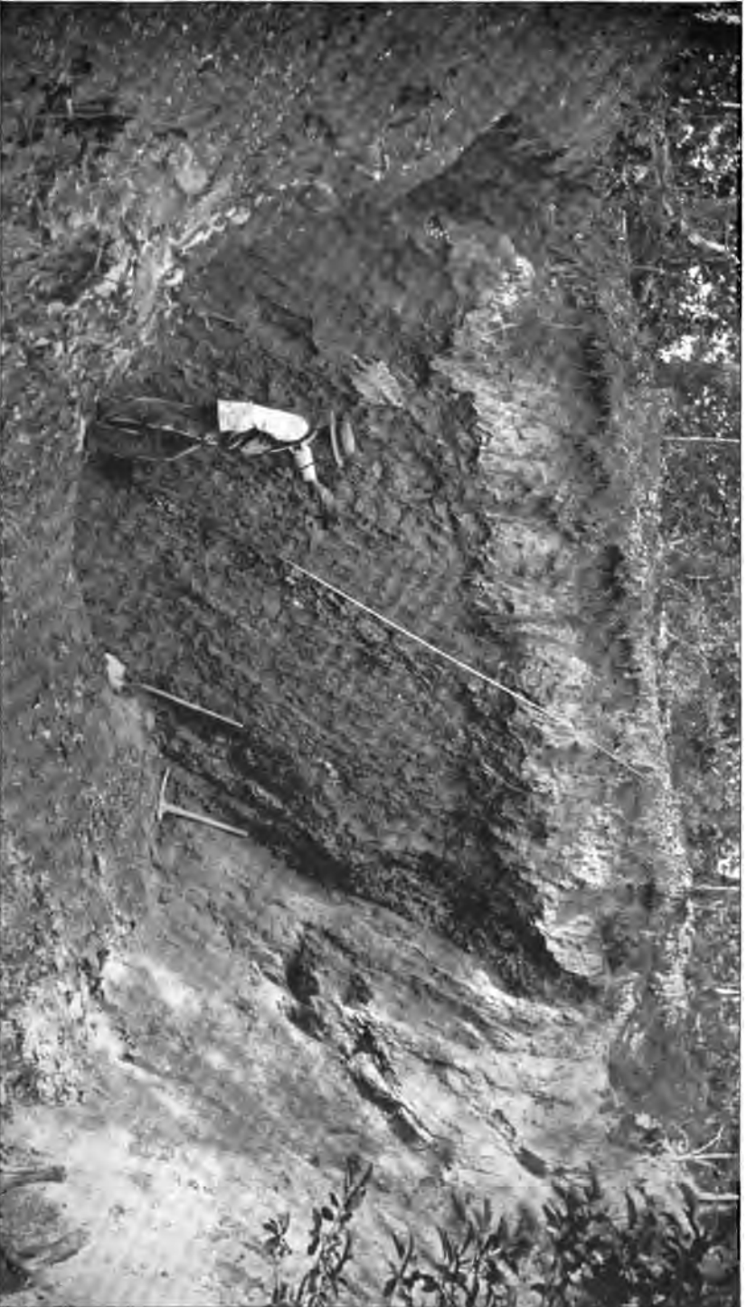
ORE-BODY IN THE MACOU MILL CUT, LA BELLE MINE, NEAR CANTON, CHEROKEE COUNTY, GEORGIA.
